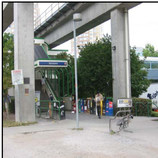
Figure 8 Existing East Station Entrance
