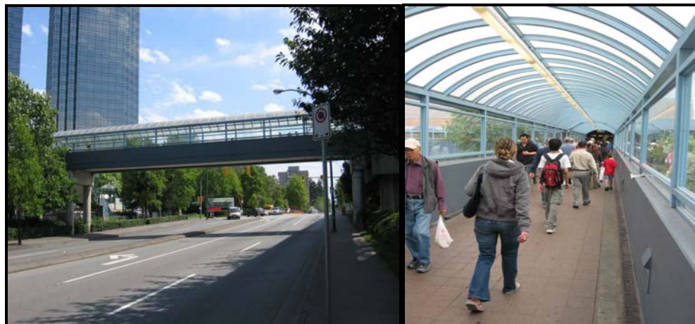
Figure 6 Existing Metrotown Passarelle
